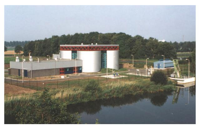
Figure 9 - Industrial water project Veendam (Groningen) with anaerobic injection water from surface water
